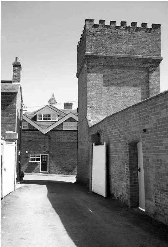
Water tower at East Langton Grange
