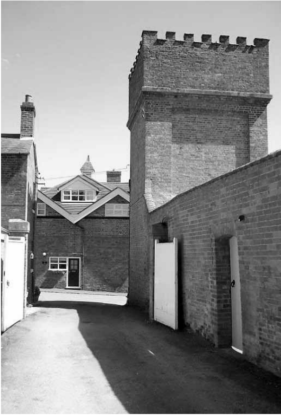
Water tower at East Langton Grange
